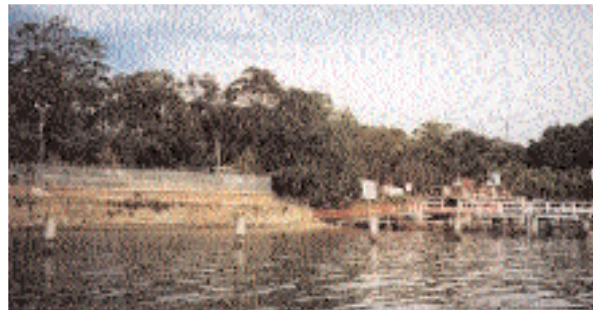
Como tidal baths are a historic example of the recreational use of Georges River, but the swimming pool cuts them off from the rest of the park.
