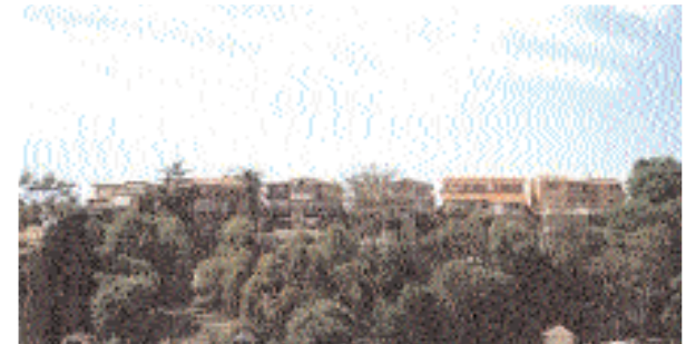
Not only do the buildings break the ridgeline but height controls have removed the sense of a varied topography.
